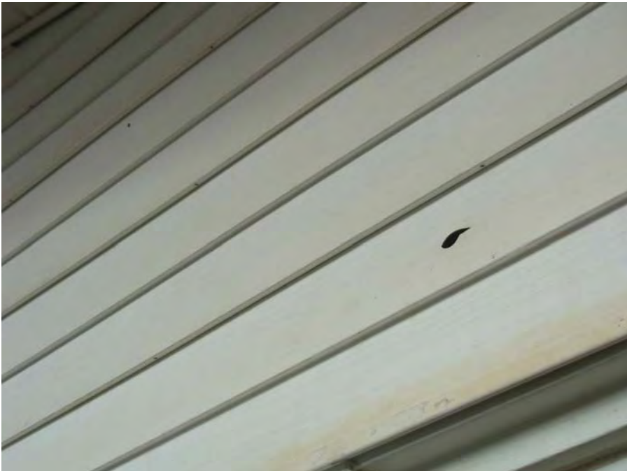
7. Spot vinyl siding impact damage
