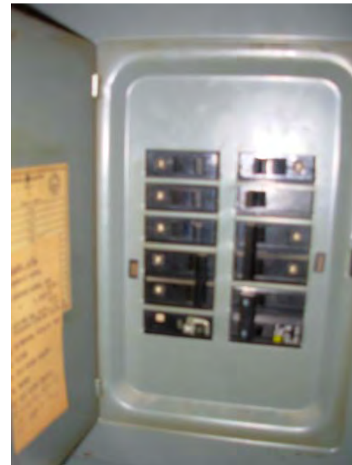
20. Original unit circuit breaker panels, to replace
