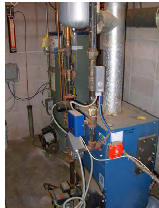
12. Heating boiler and DHW serving Cmnty. facility
