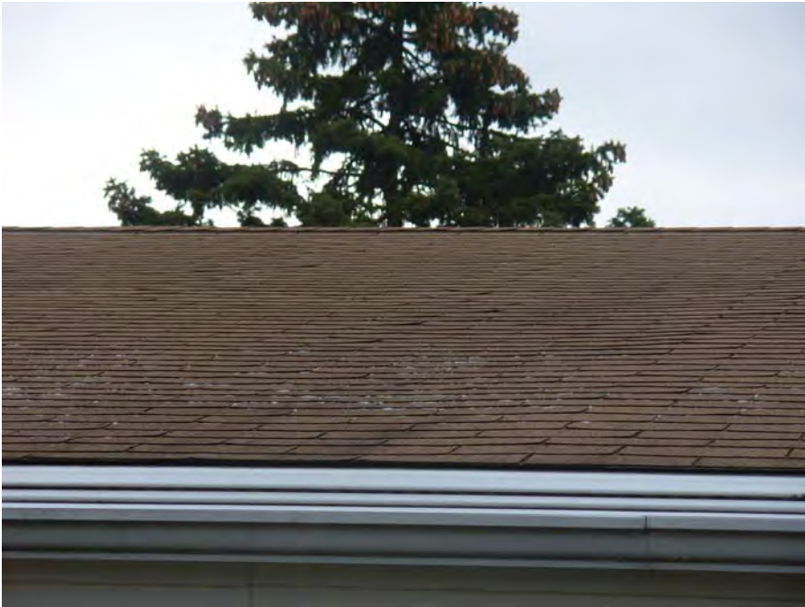
9. Spot lifting, curling of roofing shingles
