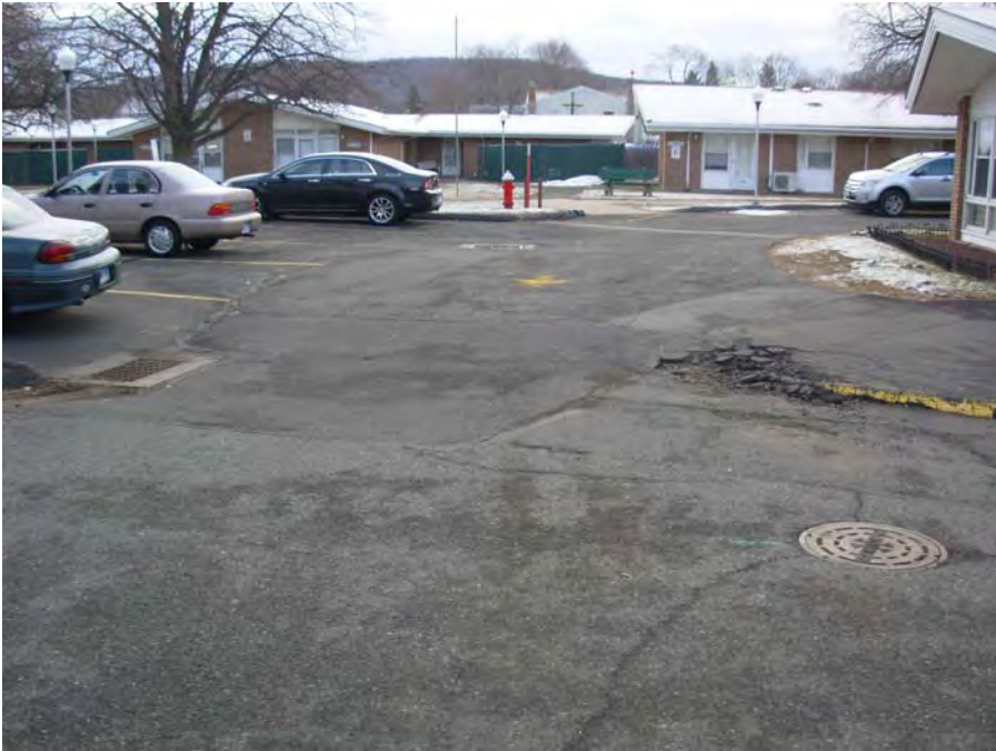
1. Site parking - paving conditions
