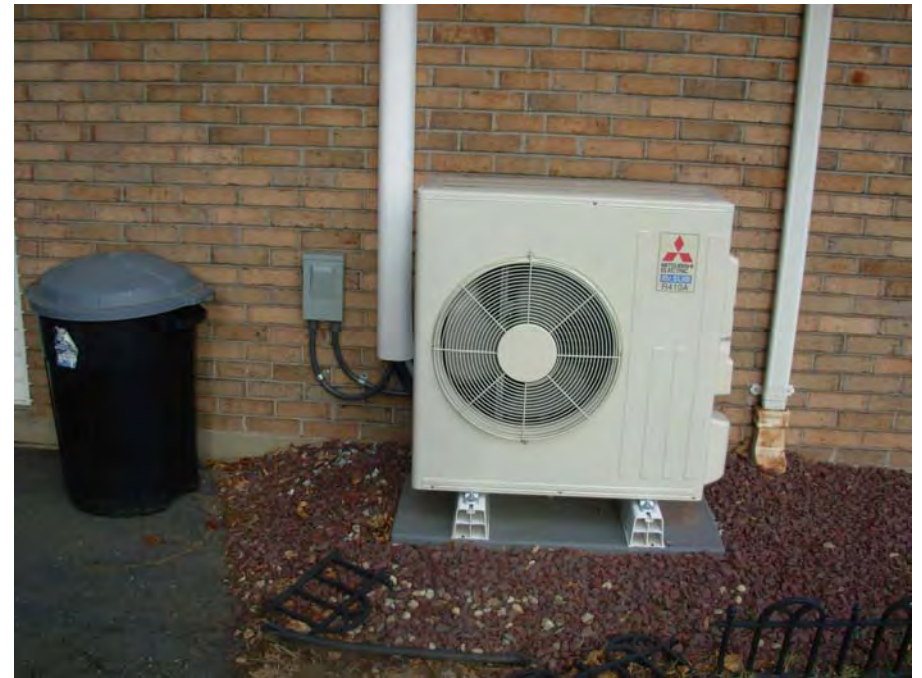
14. Typical heat pump HVAC system condenser units
