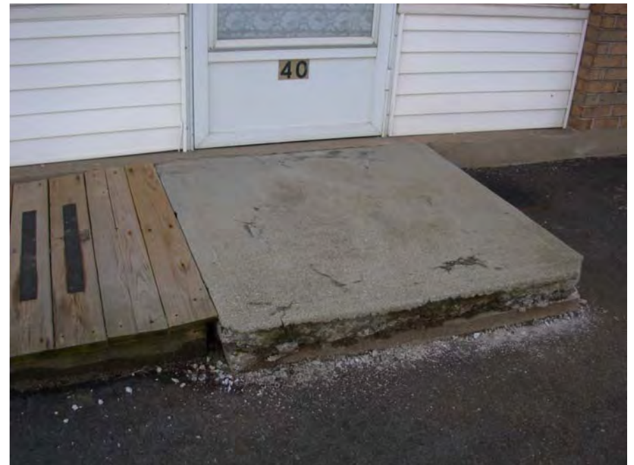
4. Some concrete spalling at stoops
