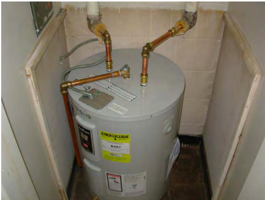
19. Electric DHW tanks serving apartment hot water needs Sunset Village • Capital Needs Assessment • © On-Site Insight
